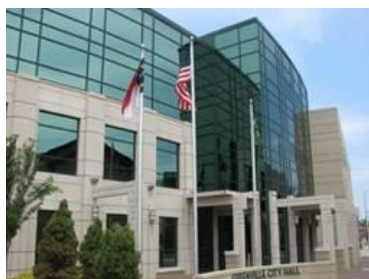
Greenville City Hall
